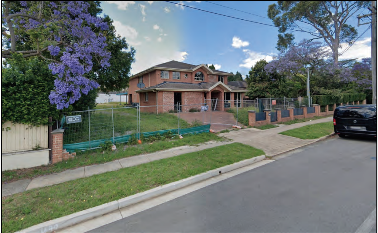
Photo 1 Existing Site at 16 Terry Road, Eastwood (Google Streetview, Nov 2021)
