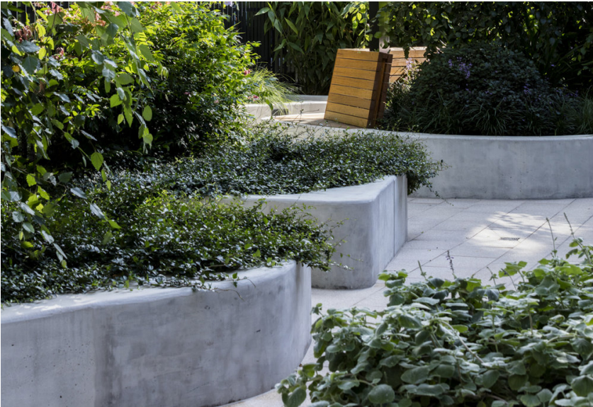
OFF FORM CONCRETE MATERIALITY
