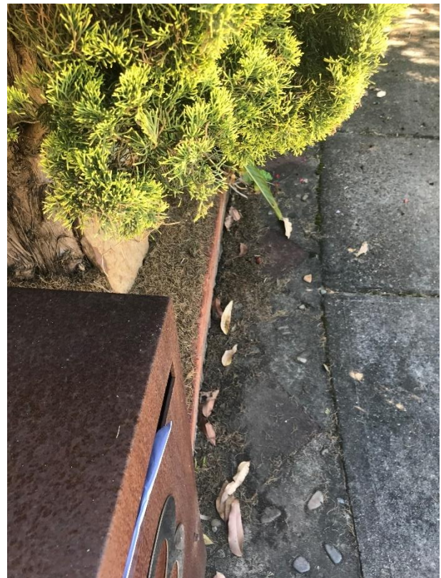
Figure 2 Tree 7 pushing front wall out of alignment
