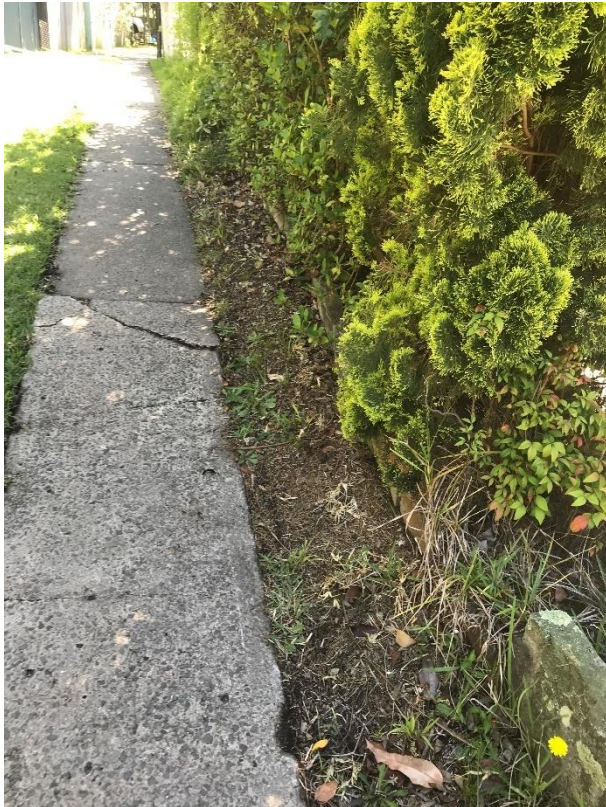
Figure 4 Tree 14 possibly causing cracking of neighbours driveway
