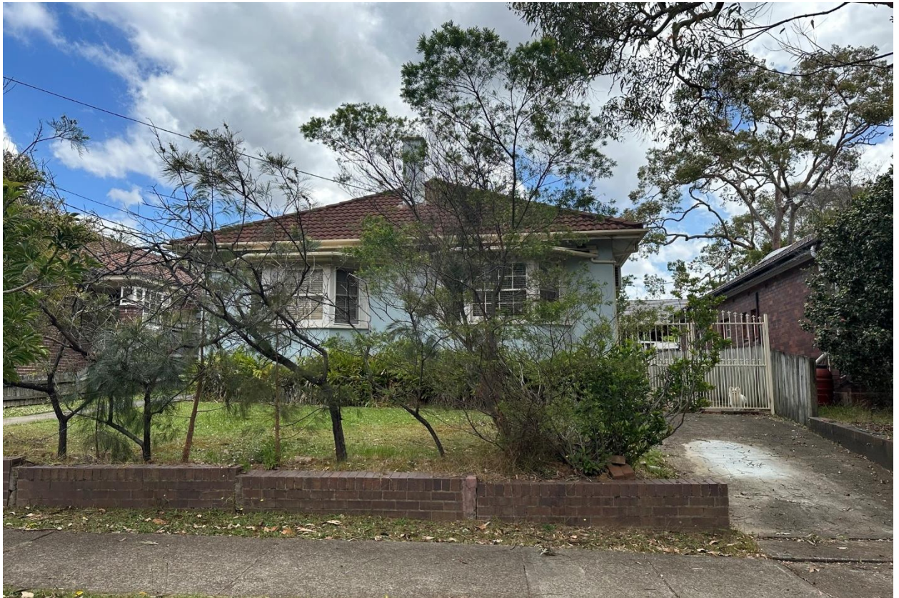
Figure 7 No. 6 Tarrants Avenue (East of the subject site).
