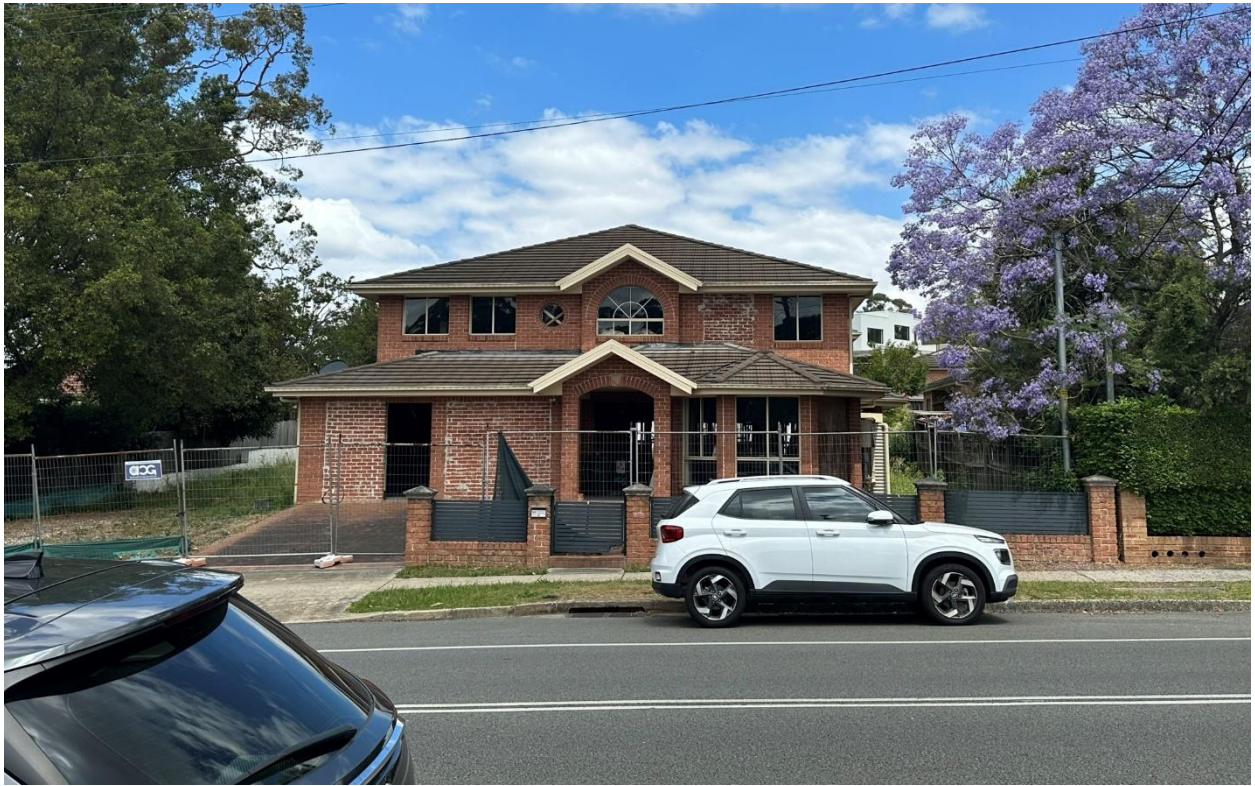
Figure 2 The subject site, as viewed from Terry Road.
